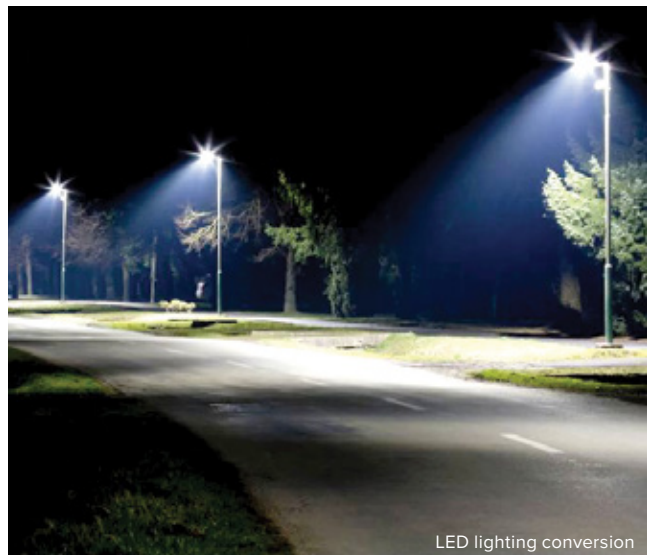
LED lighting conversion
