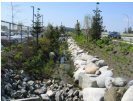
Bio-swale on North Fraser Way
