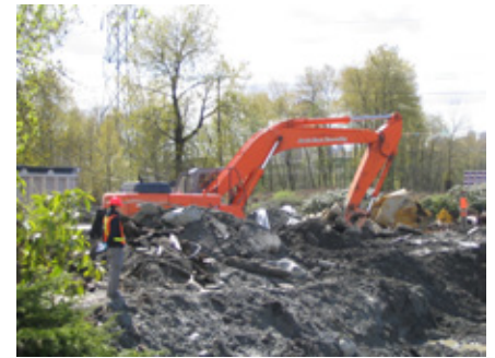
Initial preparation of creek restoration at Madison Avenue/Dawson Street development
