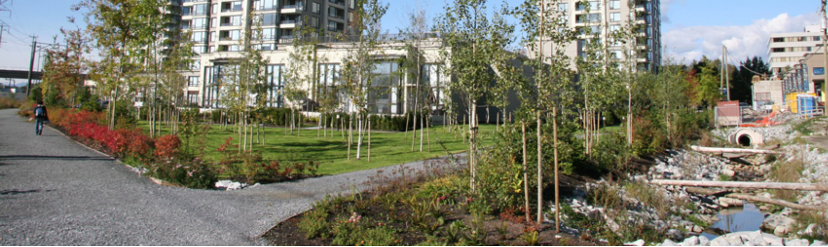
Creek restoration at Madison Avenue/Dawson Street development
