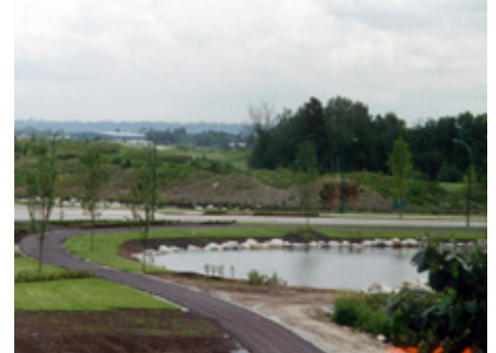
Retention pond at Glenwood Industrial Estates
