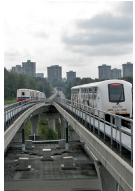
Millennium Line near Lougheed Town Centre
