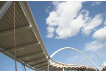
Griffiths Drive Pedestrian/Cycle Overpass
