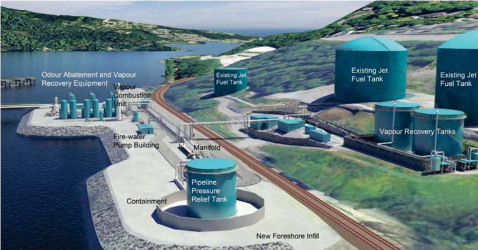
The expanded terminal would include 1.4 hectare (3.5 acres) of shoreline fill to accommodate new infrastructure
