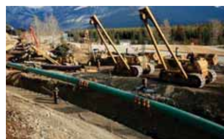
Required construction right-of-way
