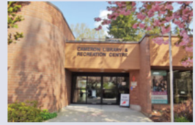
Cameron Library 9523 Cameron Street
