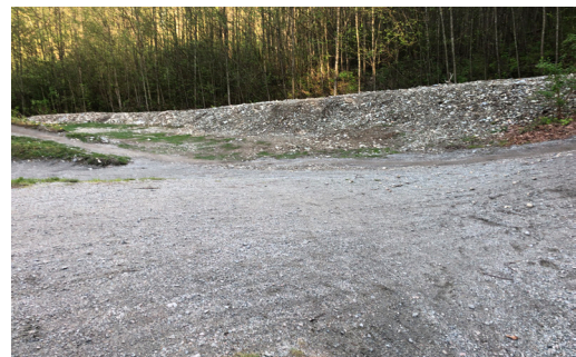
Example of gravel landings.
